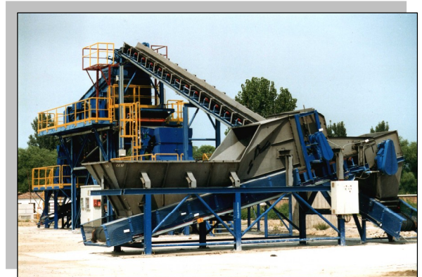
compost refining facility
